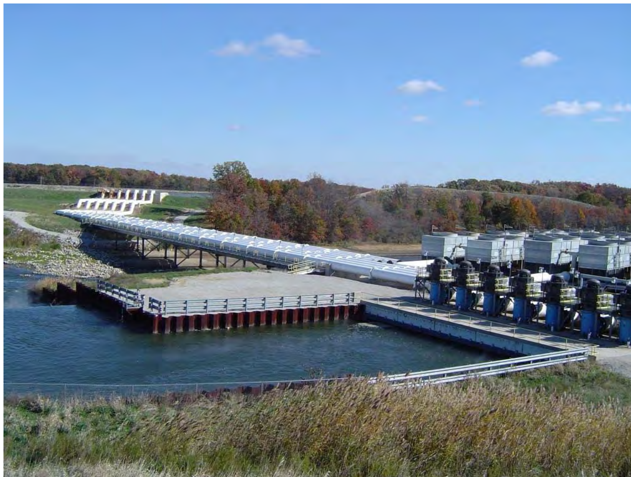
Figure 2-2. Coffeen Power Station Thermal Discharge Area Showing the 70-acre Cooling Basin (Upper Left) and 48-Cell Helper Tower (Right)
